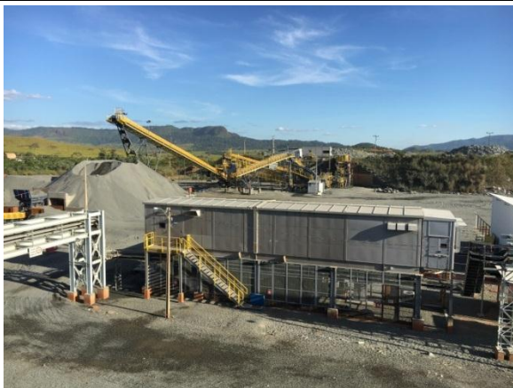
Figure 3: ROM pad, crushers & coarse ore stockpile
