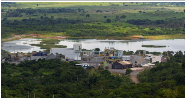
Figure 5: Processing plant and TSF
