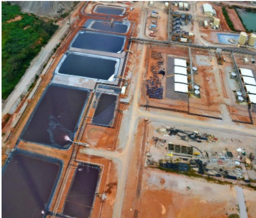
Solvent extraction circuits (high and low-grade ore) at Kinsevere copper mine, DRC. Source: www.mmg.com
